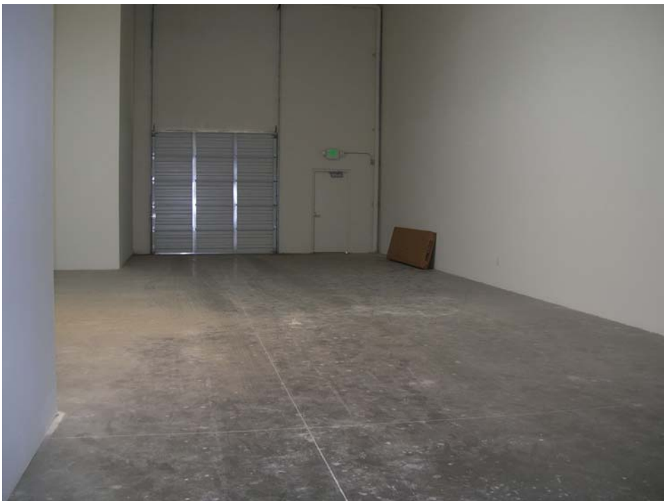
Photograph 4: Typical view of unoccupied unit – warehouse area.
